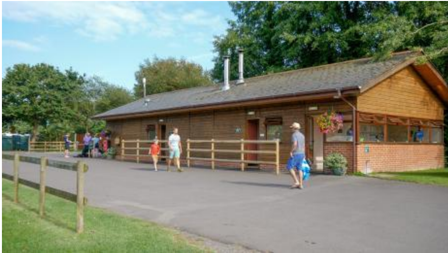
One of two Facilities Blocks
